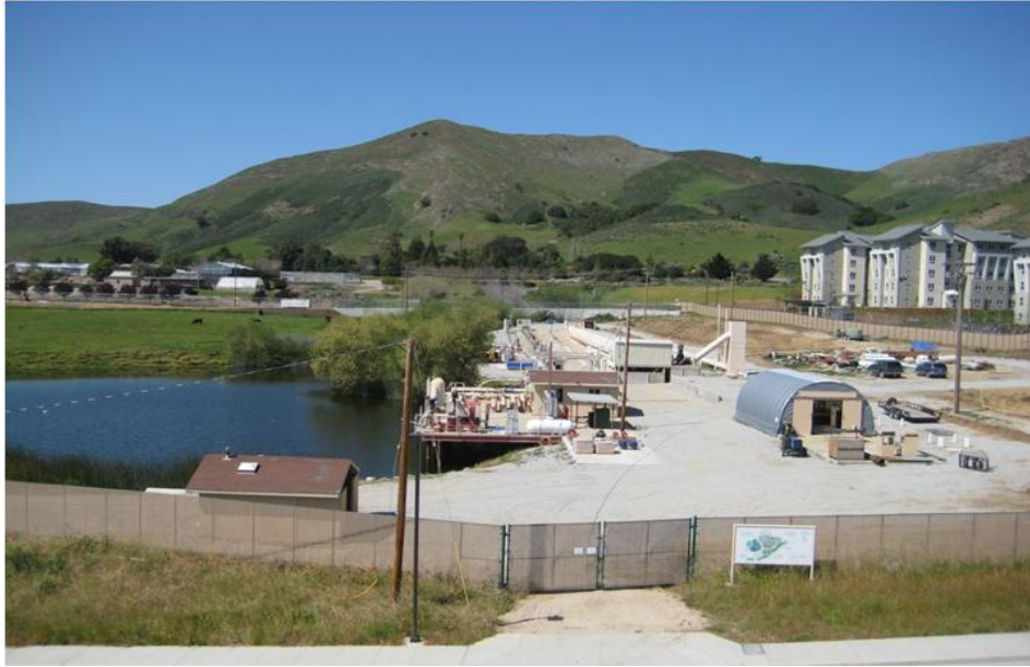
Figure 1. Cal Poly ITRC's Water Resources Facility. The flume is in the center background.
