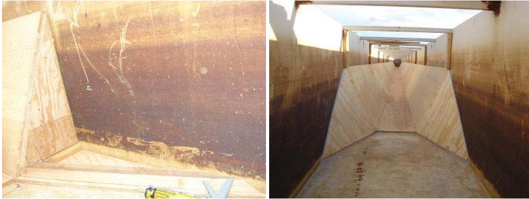
Figure 4. Cross section constructed inside the flume
