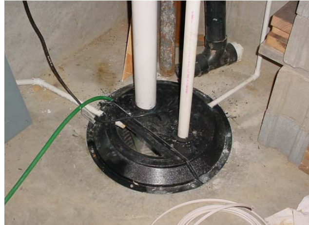
Figure 4-2. Passive sump mitigation system.
