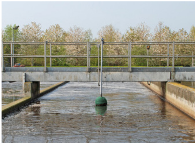
Oxix ® Ball Float solution fitted to a railing in a water treatment facility.
